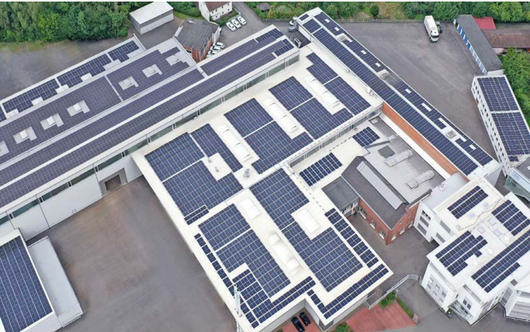
Solar modules on the company buildings: capacity increased by 81 percent.
